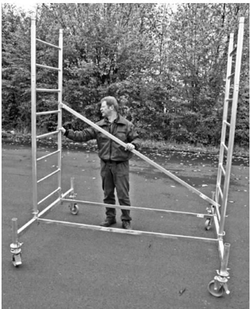
Attach the second diagonal to the fifth rung of the vertical frame to the first rung on the other side (see picture), so that it is at angles to the first brace.
